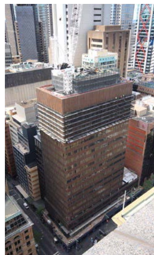
Upgrades begin at 20 Martin Place. Photo: Built
