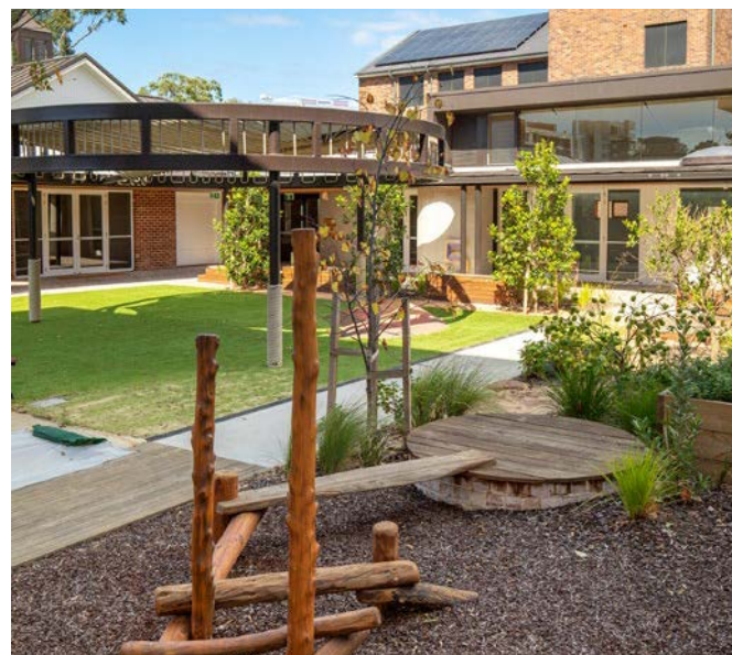
This Zetland childcare centre repurposes old hospital buildings. Photo: Katherine Griffiths / City of Sydney
